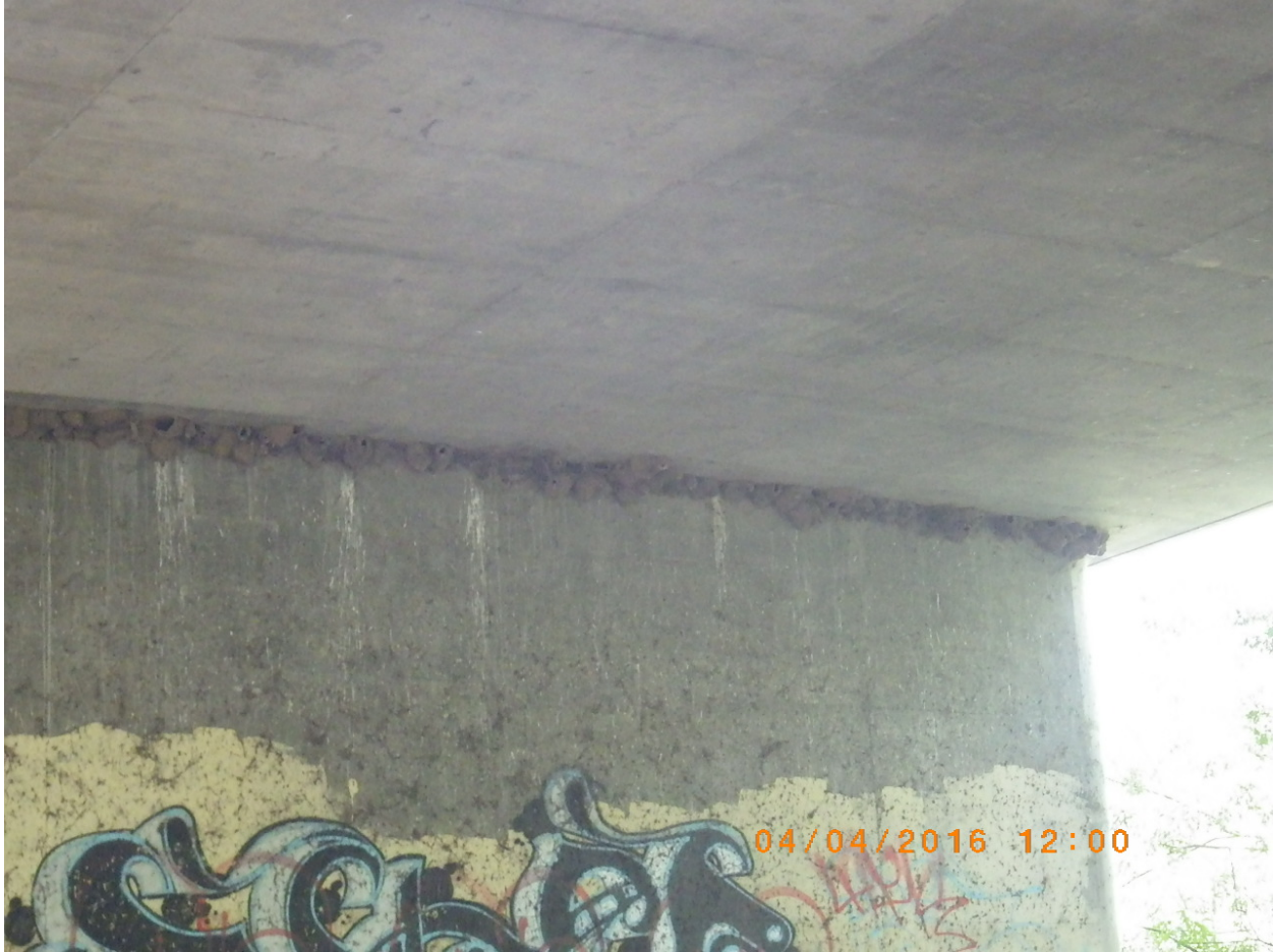
Figure 14. Swallow nests observed under a bridge at LLA
