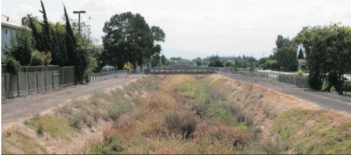
Tularcitos Creek facing South at Alcosta Drive.
