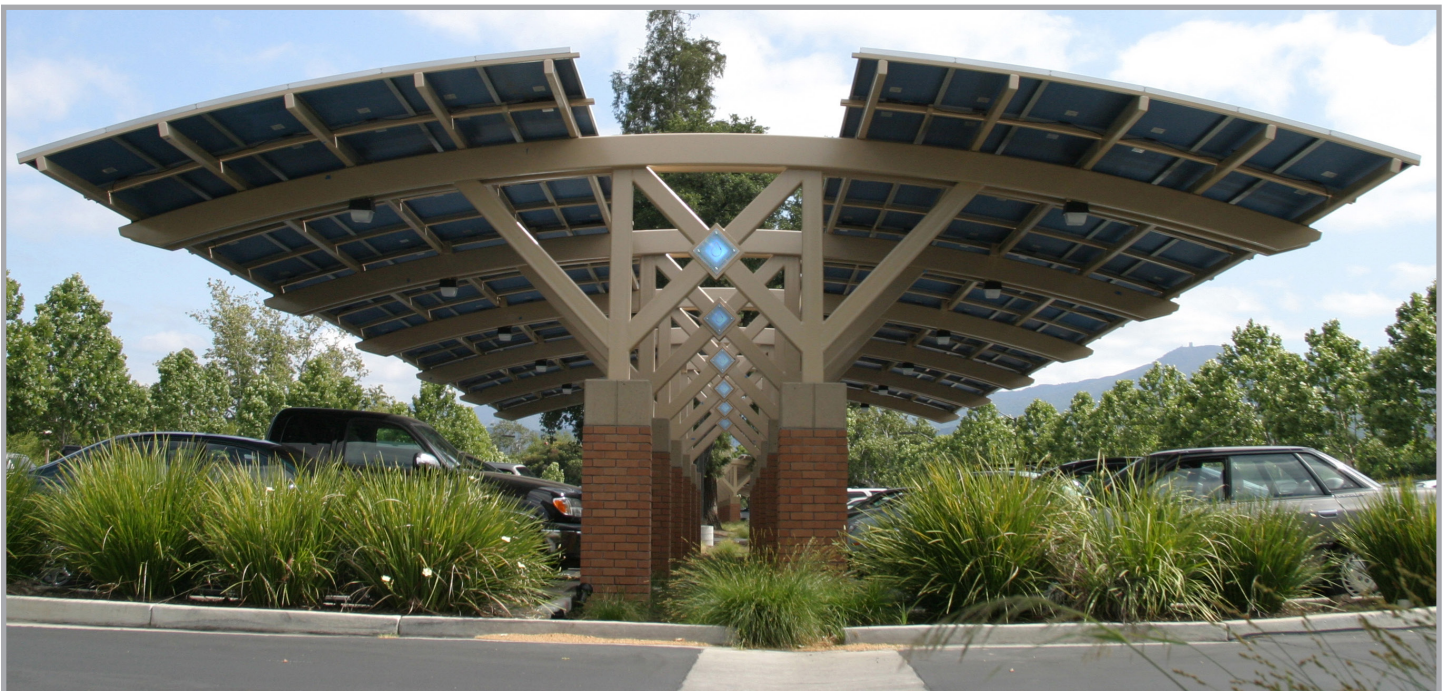
Solar panel canopies at the water district headquarters
