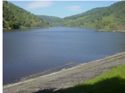
The Pacheco Reservoir Expansion Project will increase storage capacity in Pacheco Reservoir from about 6,000 AF to over 140,000 AF.
