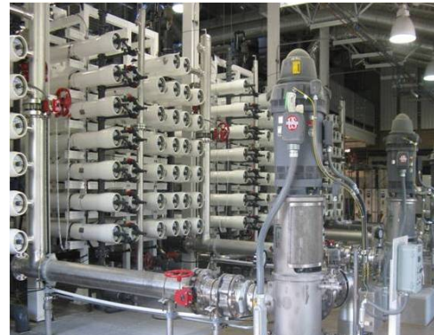
Reverse osmosis is one step in the advanced treatment process for purified wastewater.
