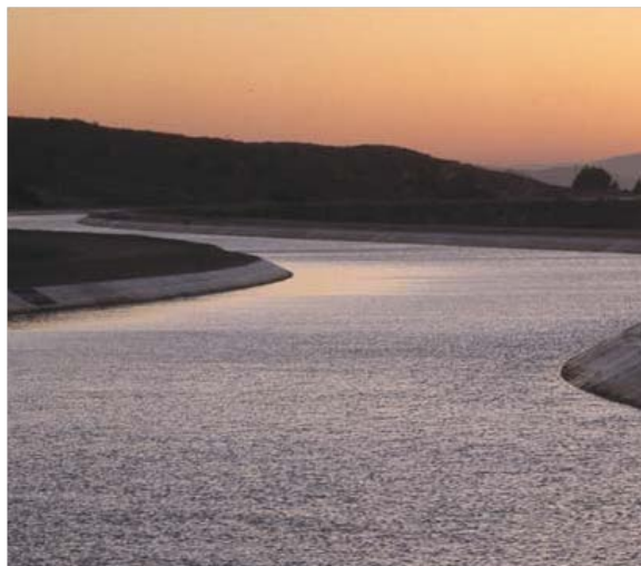
The California Aqueduct delivers Delta-conveyed supplies to municipal, industrial, and agricultural customers
