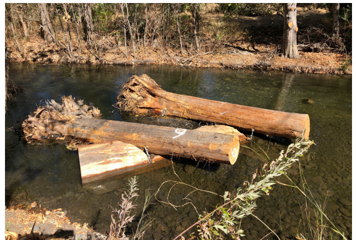
Installed Large Woody Debris.
