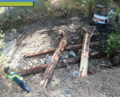
Crews will install anchored logs into the Los Gatos Creek. Strategically placed logs can give fish places to rest and evade predators.
