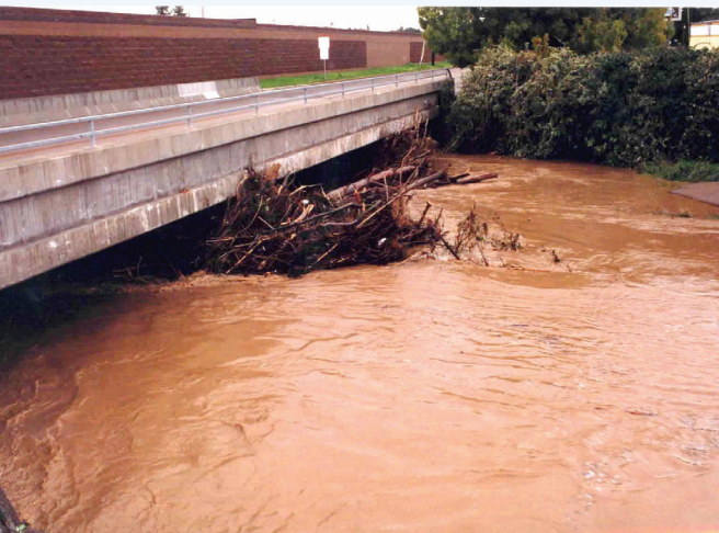
The 1998 flooding of San Francisquito Creek closed Highway 101 and caused an estimated $28 million in damages.
