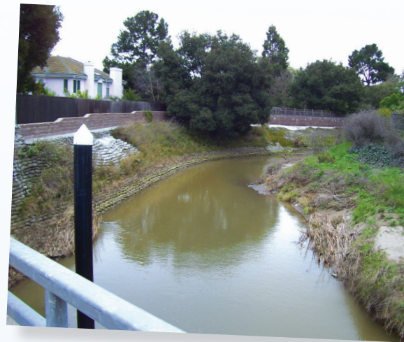
A debris deflector protrudes up from beneath the Bayshore Freeway bridge, where it prevents the accumulation of flood debris that can block water flow and cause flooding to nearby homes. The facing page photo shows debris accumulating at this same bridge before the deflector was installed.
