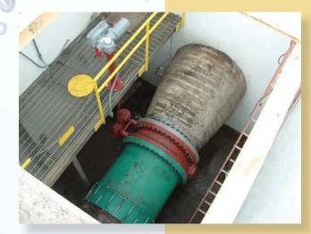
New line valves will allow the District to isolate sections of pipeline during repair and maintenance, which will reduce the risk of outages after a major earthquake.
