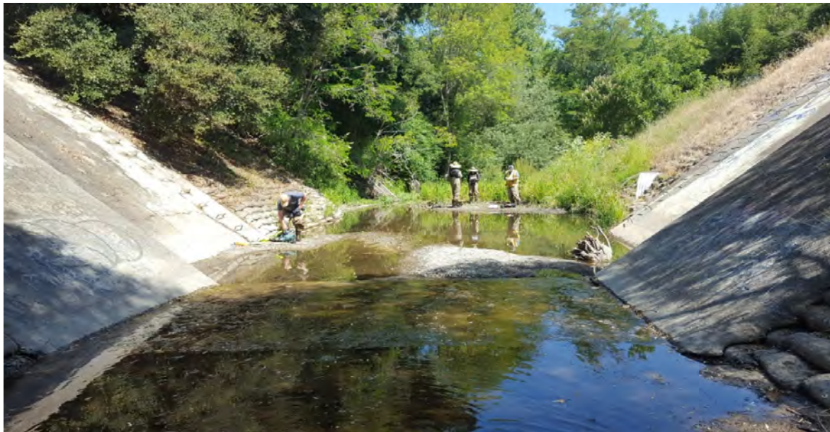
Looking downstream from above drop structure and concrete channel bed
