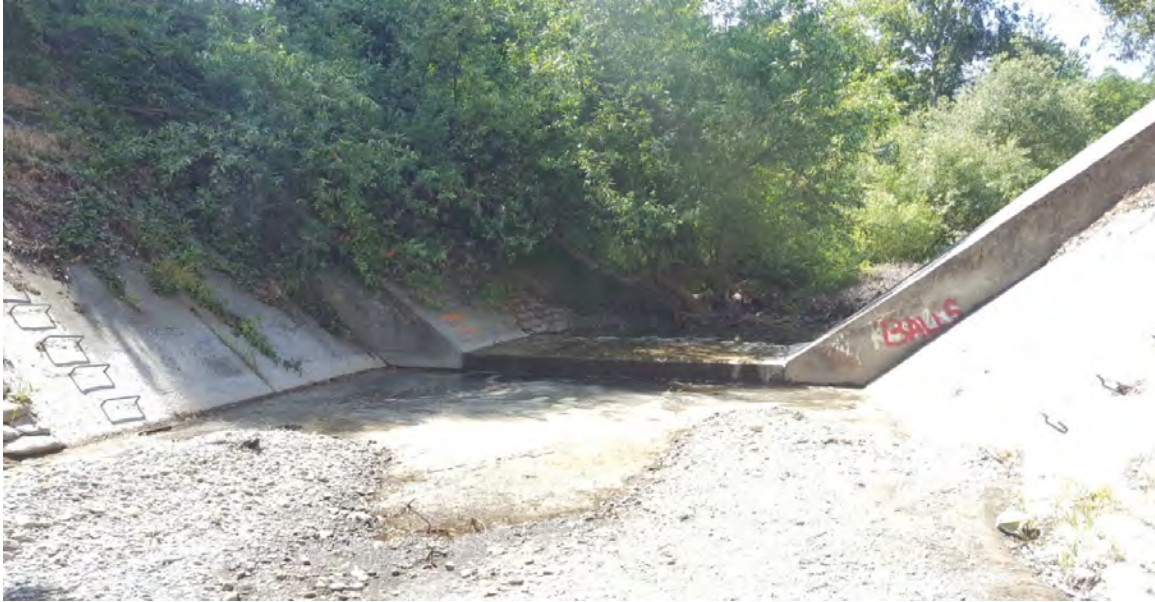
Looking upstream to drop structure
