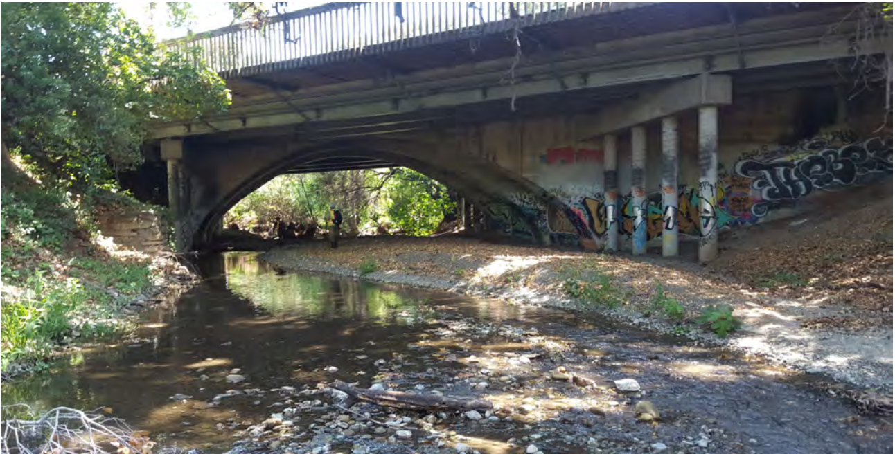
Culvert outlet facing upstream
