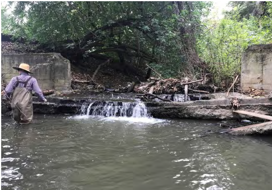
Drop structure looking upstream from scour pool
