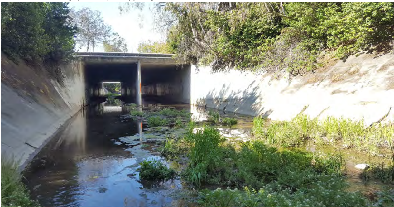
Culvert outlets looking upstream, primary passage culvert on left
