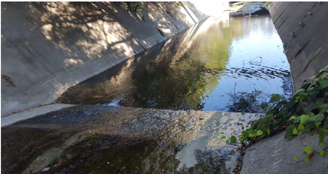
Looking downstream from top of drop structure
