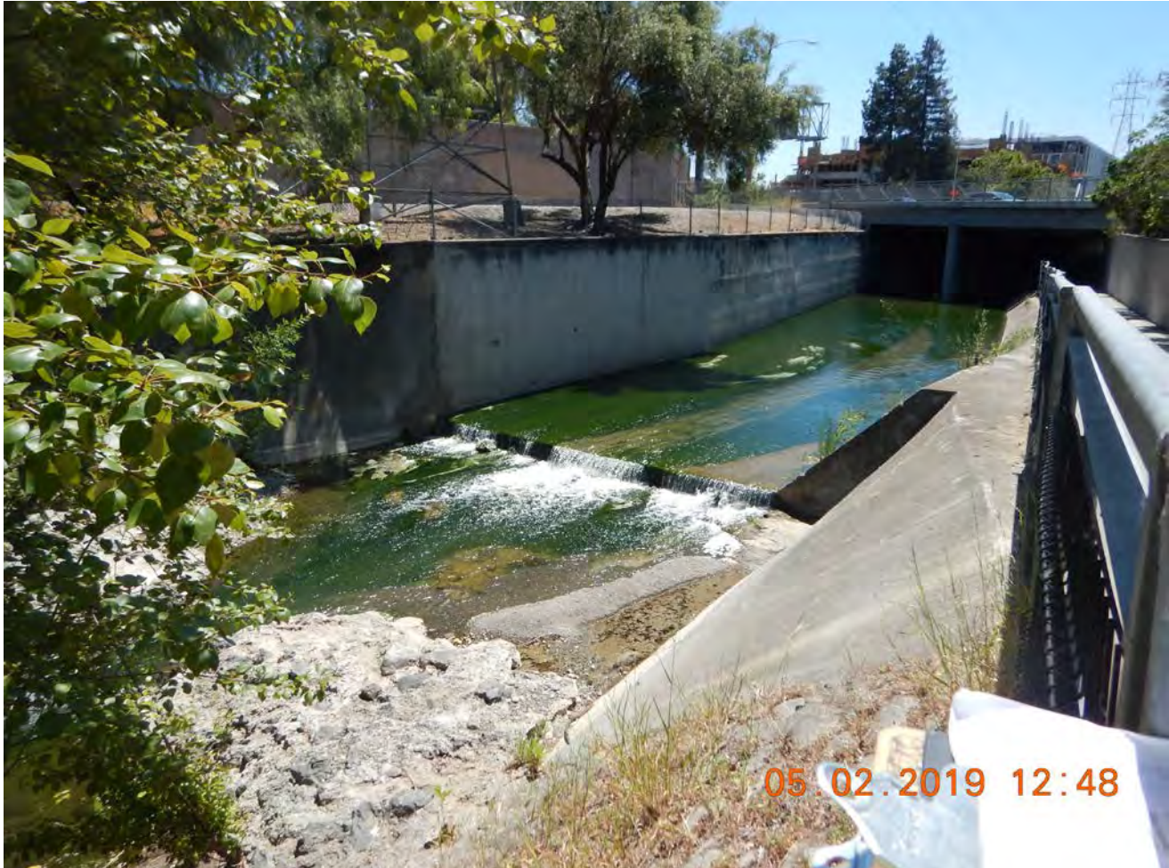
Photograph 3: Highway 101 culvert and chute
