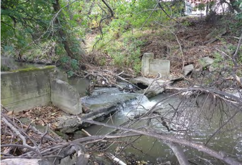
Drop structure looking upstream from right bank
