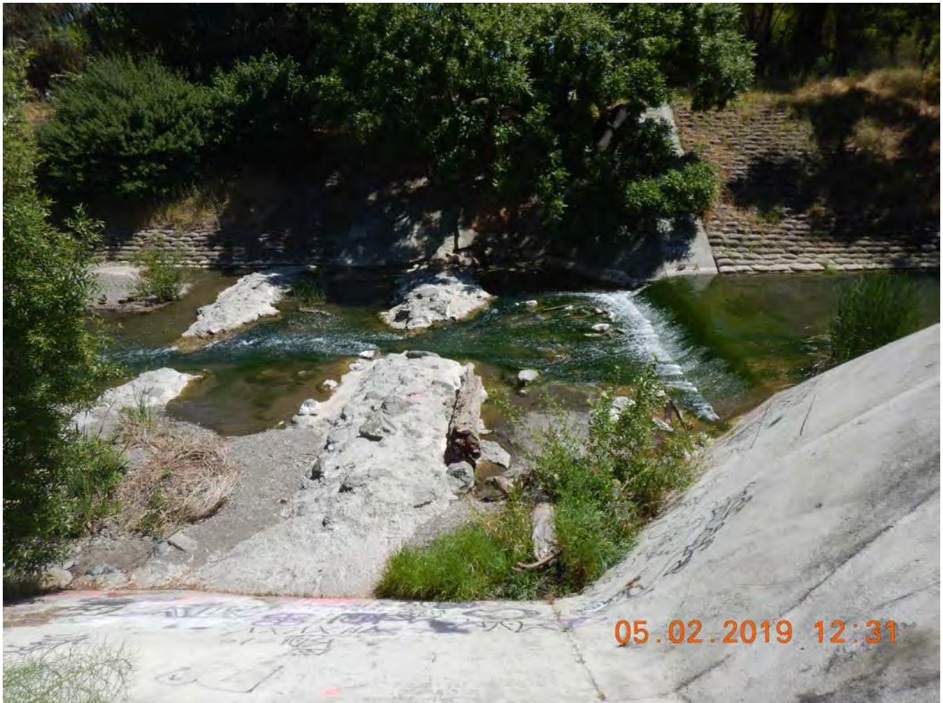
Photograph 4: Grade control structure at Vernon Avenue
