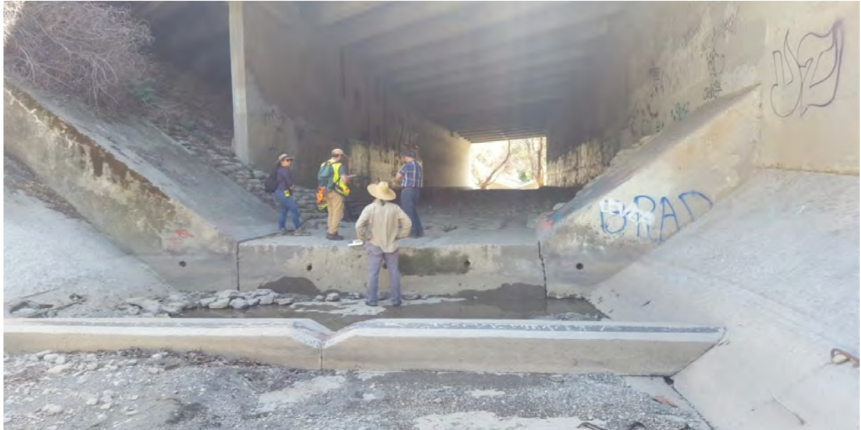
Looking upstream to drop structure and bridge, with v-weir in foreground
