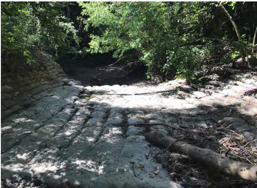
Looking downstream at drop structure/drainage outfall protection
