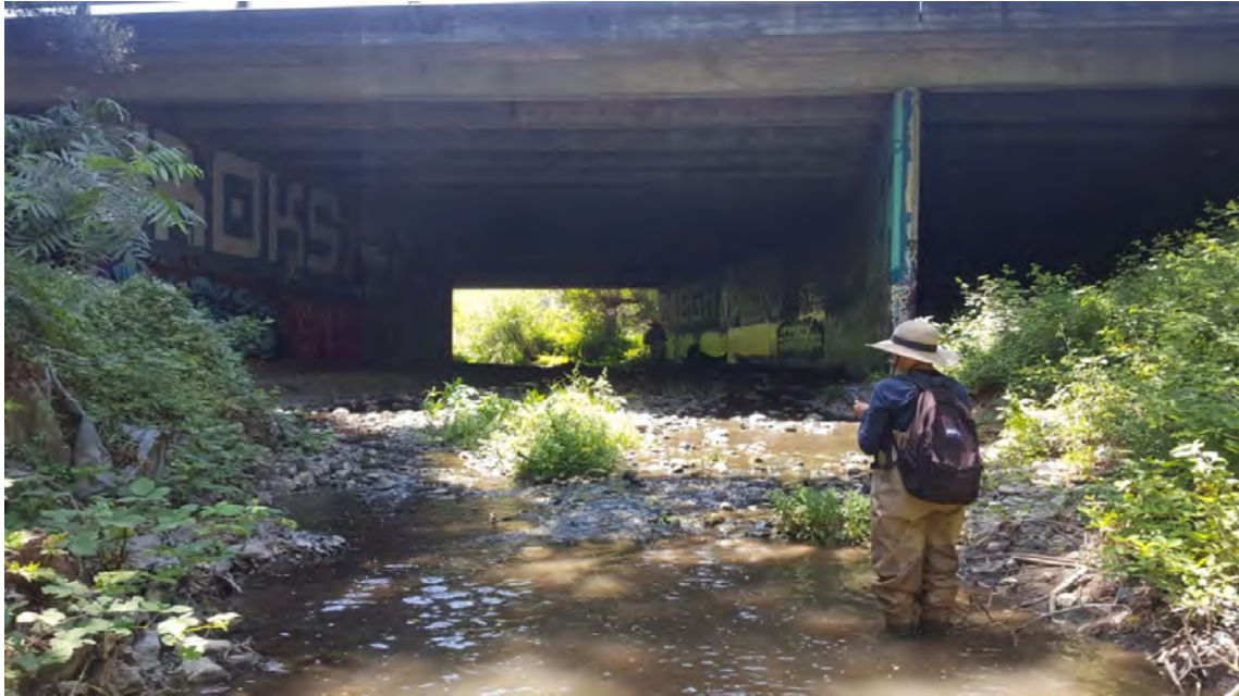
Bridge outlet looking upstream
