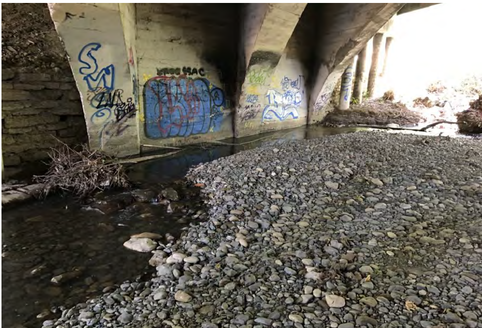
Inside culvert, facing upstream
