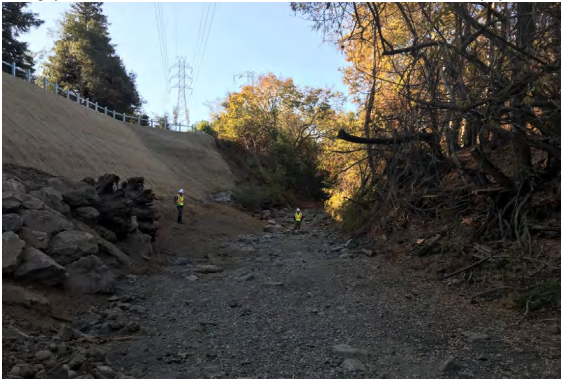
Looking upstream at downstream end of boulder channel and 2018 bank stabilization project
