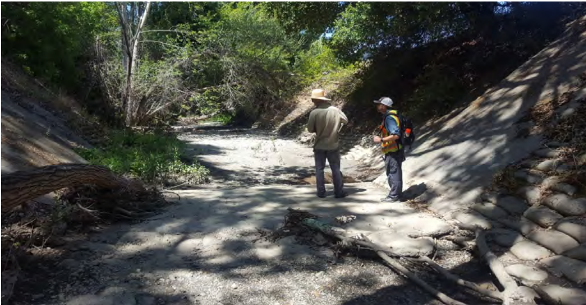
Looking downstream from above drop structure
