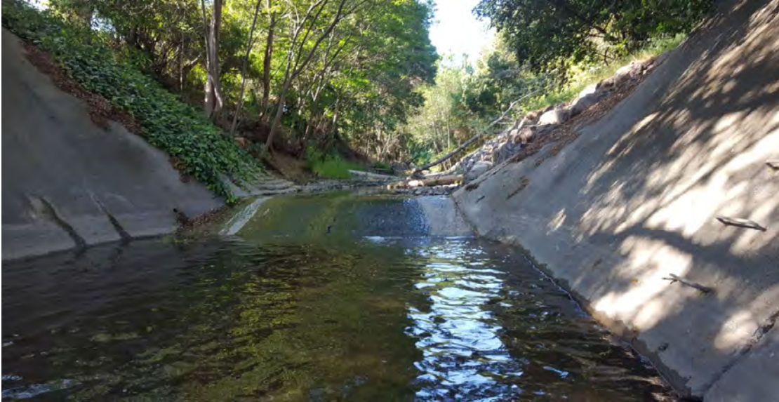
Looking upstream to drop structure
