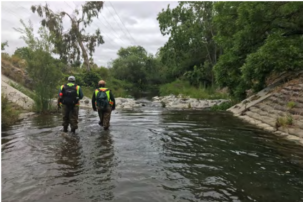
View from upstream looking downstream at drop structure
