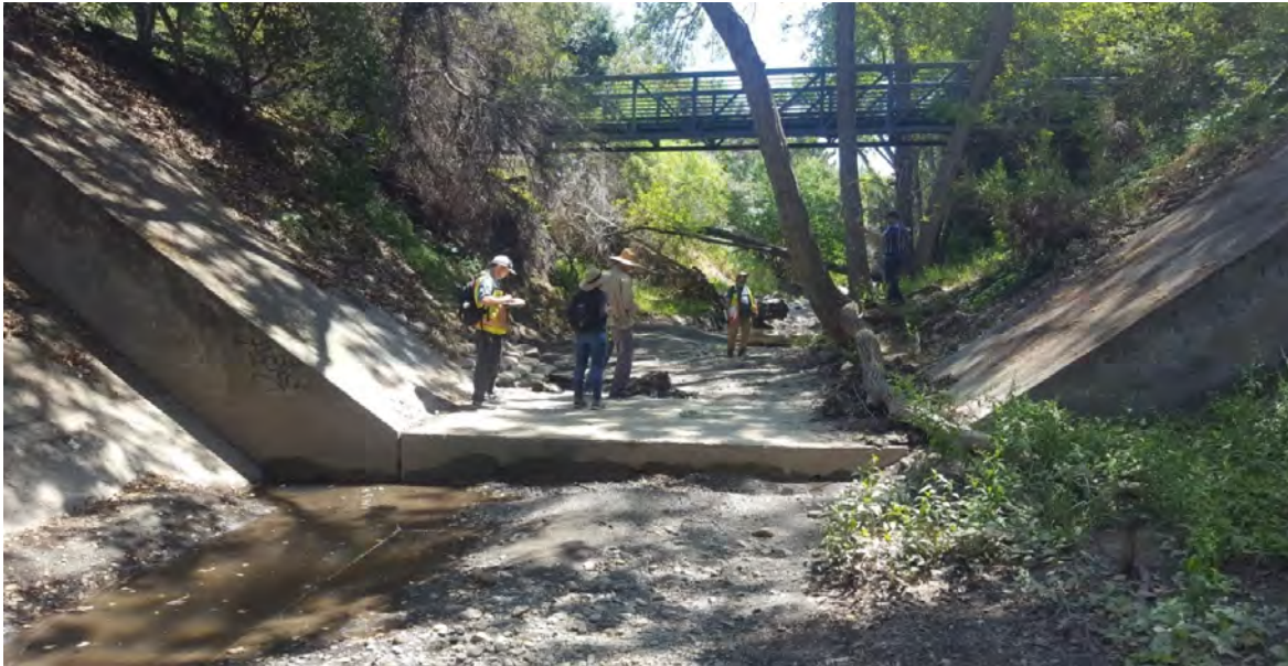
Looking upstream to drop structure
