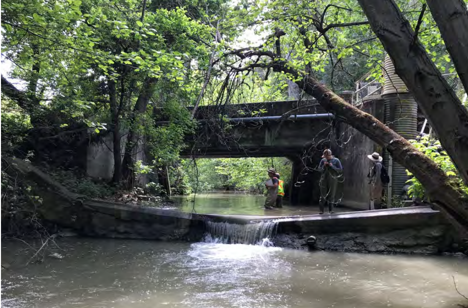
Looking upstream at riffle control of pool below gaging weir
