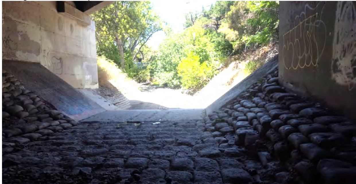
Looking downstream to drop structure from within culvert with sacrete invert
