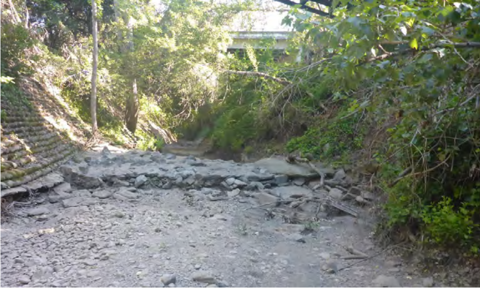
Grouted boulder drop structure looking upstream
