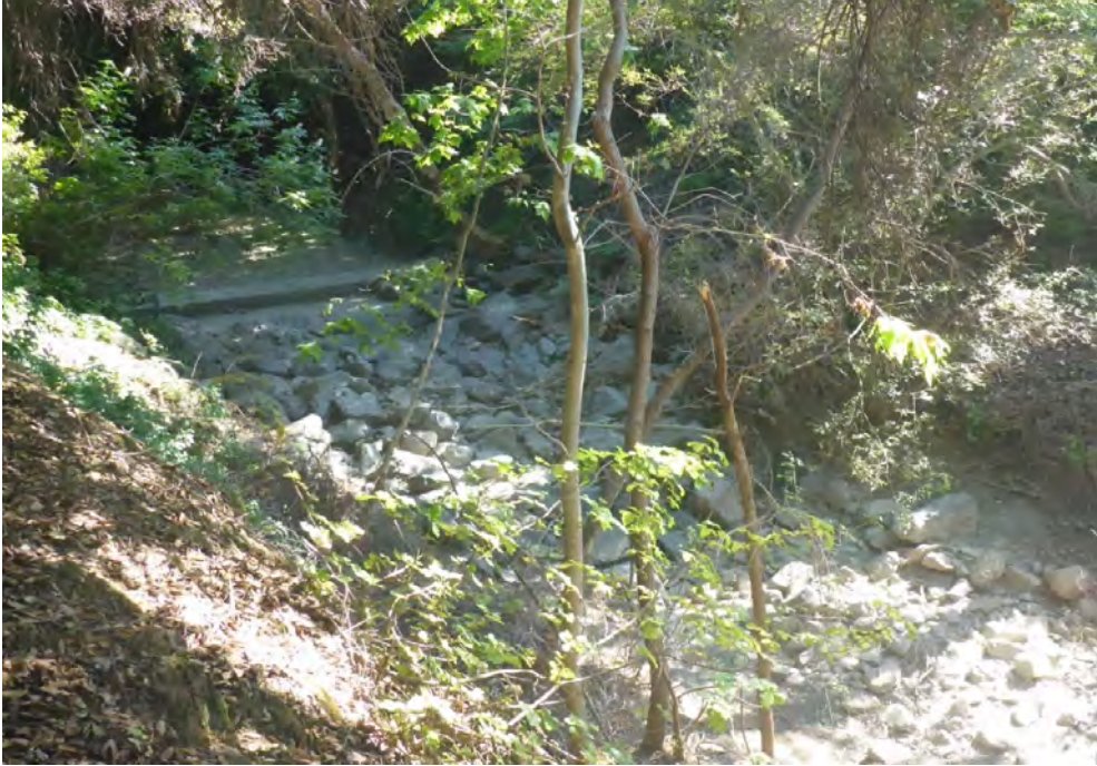
Concrete grade control with boulder chute below, looking upstream
