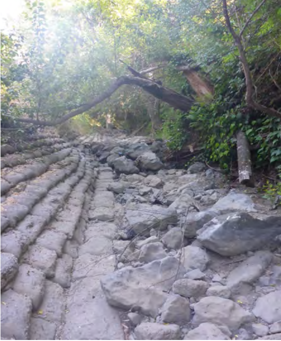
Looking upstream at boulder jam
