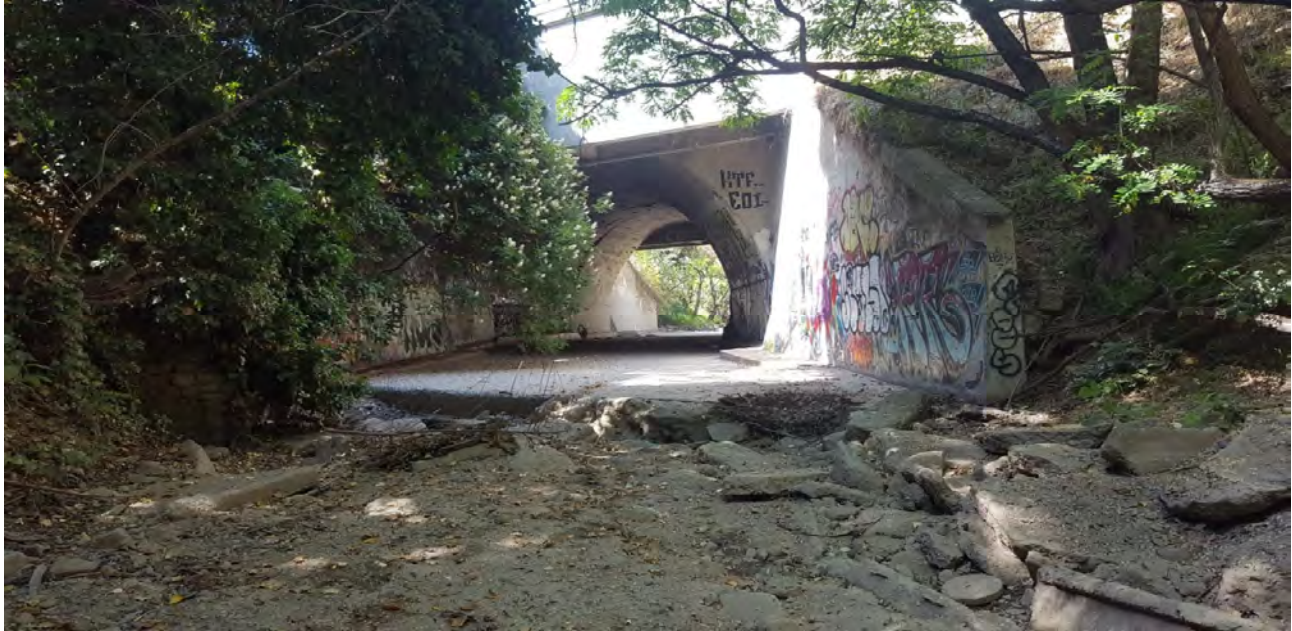
Looking downstream at culvert inlet
