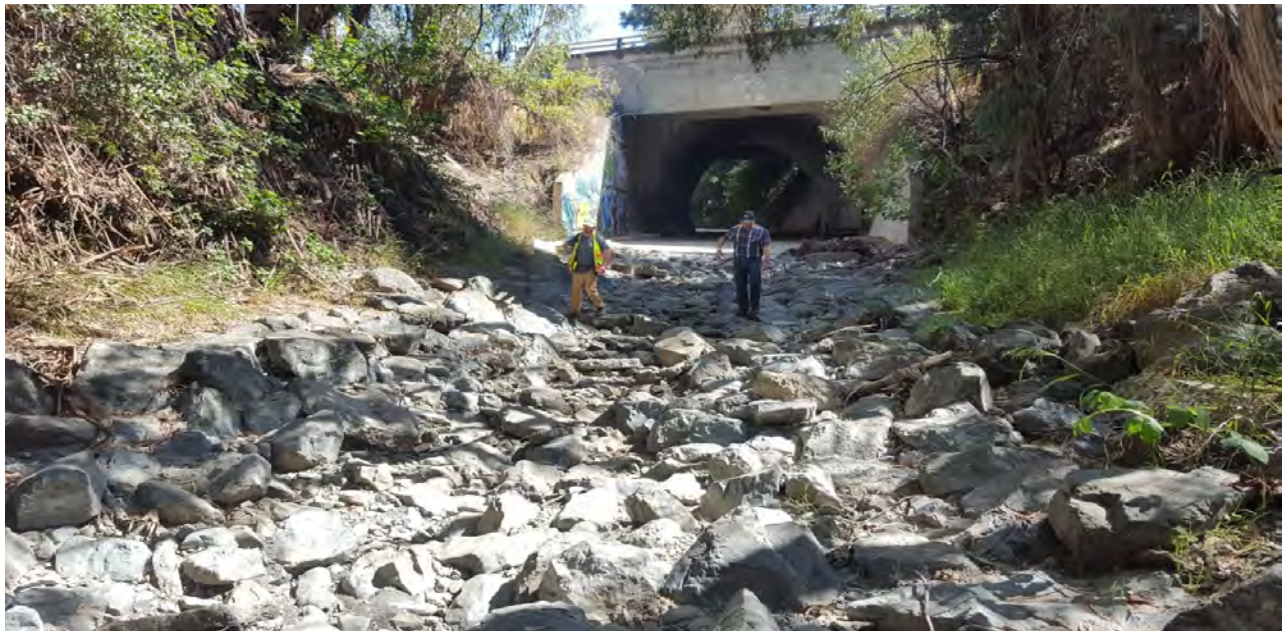
Looking upstream at culvert outlet with boulder channel (site 16) downstream of apron
