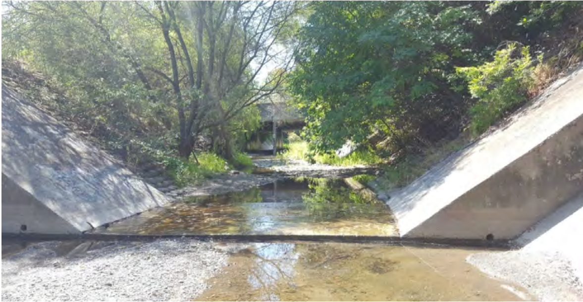
Looking upstream to drop structure
