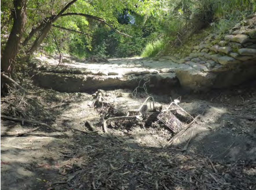
Looking upstream at drop structure/drainage outfall protection
