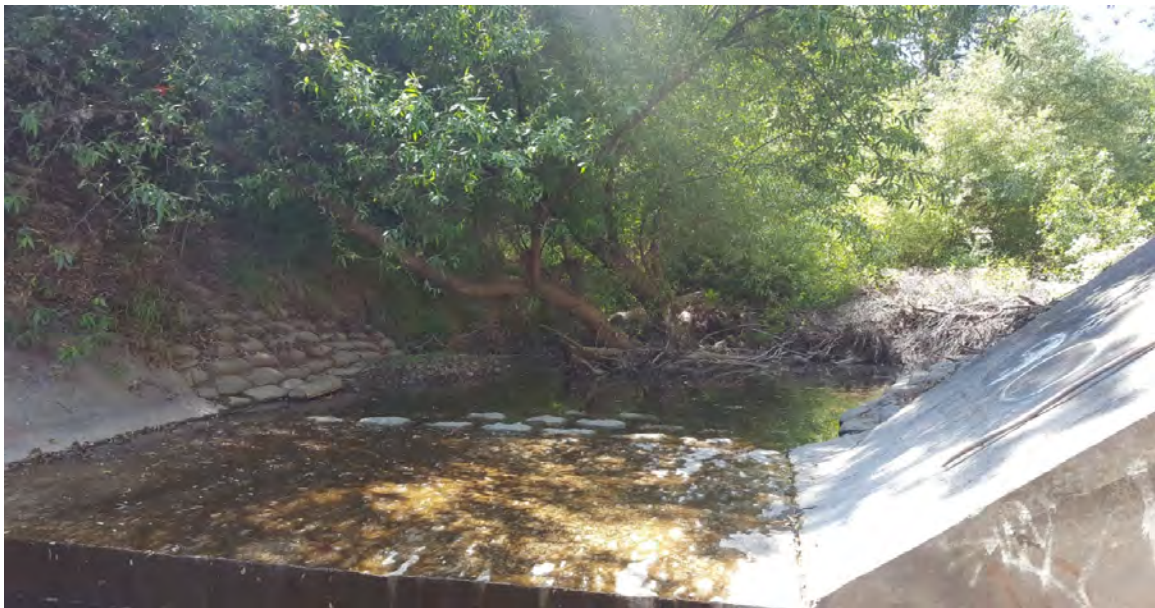
Looking upstream to above drop structure
