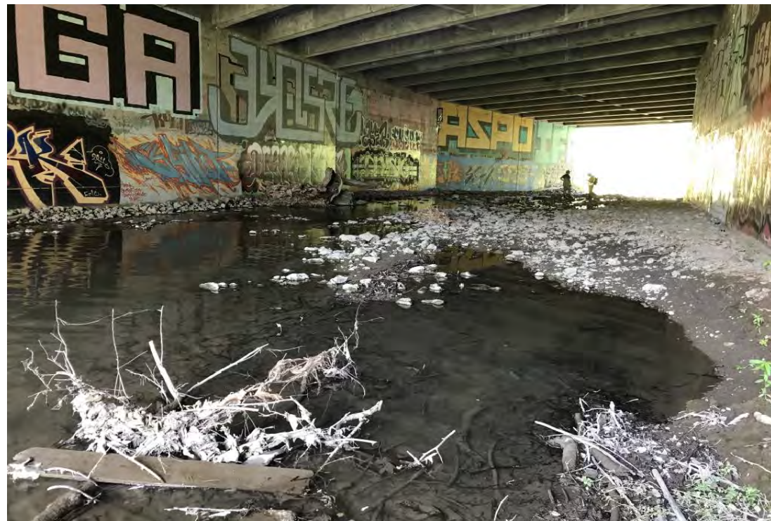
Inside bridge, looking downstream.
