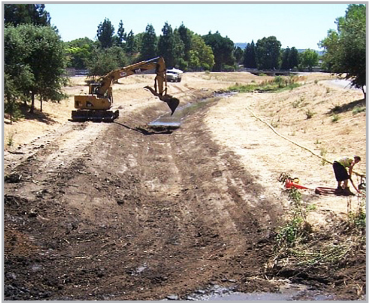
Most project construction activities will involve creek channel deepening and widening work as shown above.
